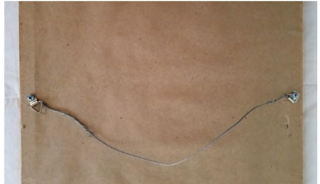
Kraft paper dust cover with v-ring and wire in place.
